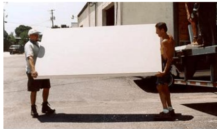
Exterior Wall Section Weights 38 Pounds
